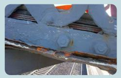
One of the main challenges is station footbridges; there is often a need to erect an alternative footbridge when the existing one is under repair, as the repairs usually take a long time for a variety of reasons. With a number of structures under deconstruction, the hidden critical elements are found to be in a poorer state than previous thought and therefore, the remediation that had been proposed is no longer fit for purpose.
